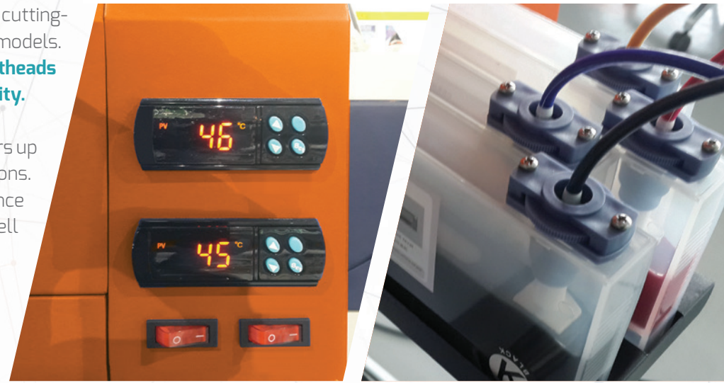
Heater temperature controllers
